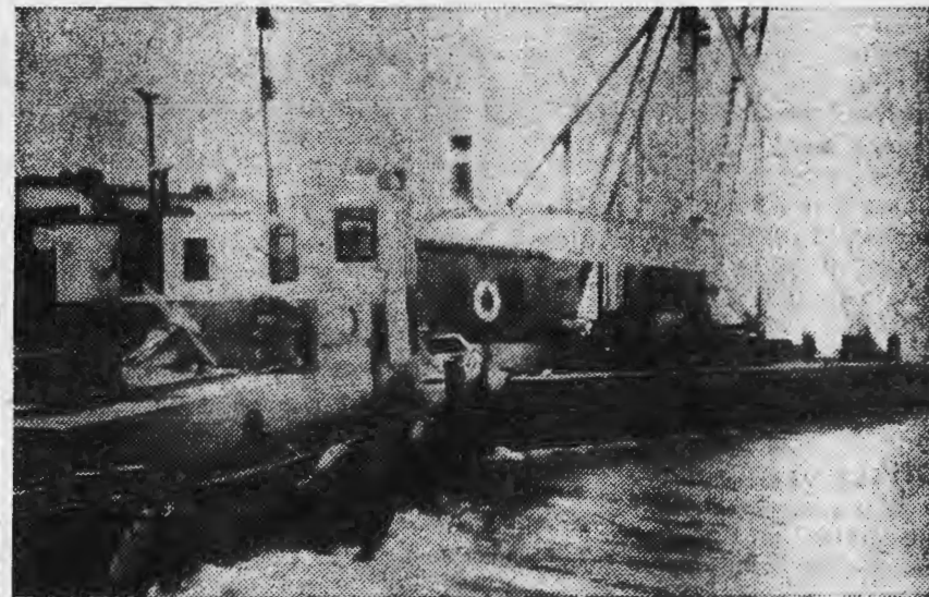
Picton's derrick-barge Roberts is pictured while idle during IBU strike, before she was scabbed out by a tug manned by members of National Maritime Union affiliate. The derrick was towed to dredge job in Louisiana.
