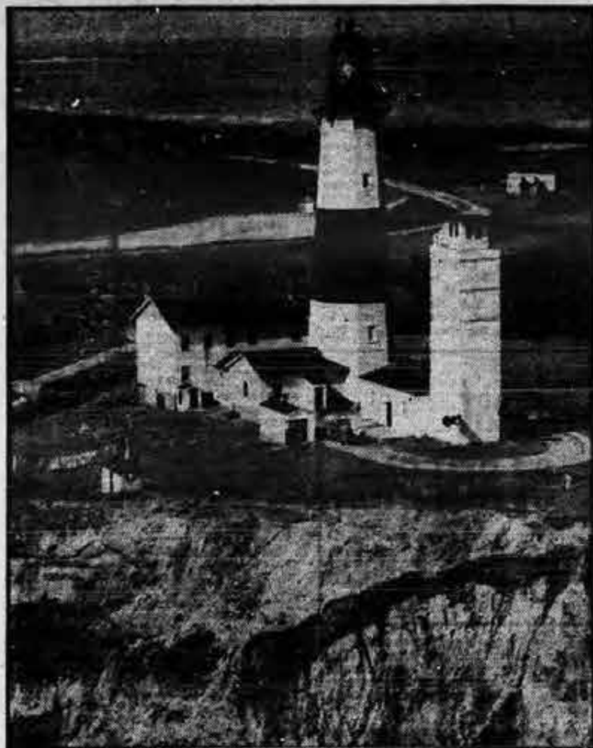
Dating back to Washington's time, famed Montauk Light is menaced by the sea, with steady erosion of the cliff on which it rests. The sea is now barely 100 feet from the lookout tower in front of the lighthouse itself.
