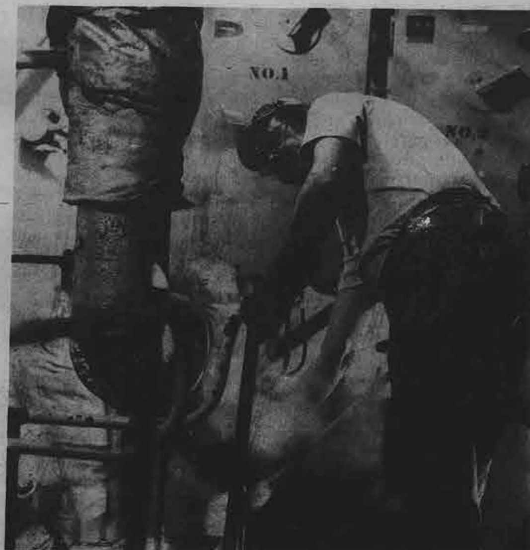
Oiler Larry Mays fights off steam in the engine room of the tanker Overseas Valdez as he starts up cargo pumps. The ship was in the port of New York recently lightering at Stapleton Anchorage off Staten Island, N.Y. Larry's got plenty of seafare under his belt having been a member of the SIU since 1952 and in the Navy for seven years before that. A native of Hamilton, Ala., Larry now makes his home in Houston, Tex.
