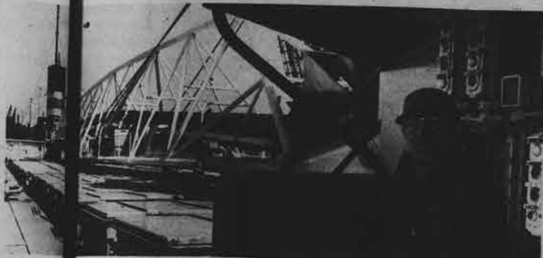
Conveyor operator Lenord Arendt tests the Nicolet's equipment and finds everything to be in ship shape. The new self-unloading crane takes up almost all of the vessel's deck space.
