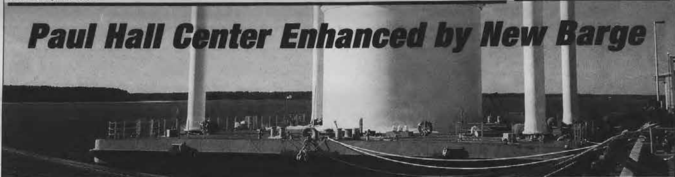
Now moored in Piney Point, the Empress II still features part of the pulse generator/antenna system once used to simulate electromagnetic pulses.
