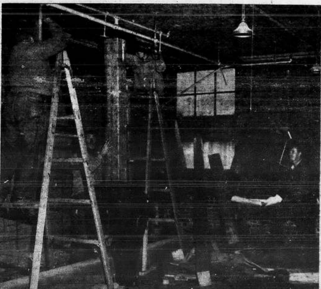
Work is proceeding smoothly on the renovation job begun last week on the SIU's new Headquarters-Port of New York building. Here workmen are shoring up the overhead preparatory to knocking down bulkhead that will enlarge first-floor area to be occupied by the cafeteria. Frenchy Michelet (extreme right), who is supervising the alteration work for the Union, looks on. When this section is completed the cafeteria will be large enough to seat more than 250 persons at one time. Located on Fourth Avenue, between 20th and 21st Streets, Brooklyn, the new Hall will give Seafarers a fully-equipped, modern structure with increased facilities for membership services.
