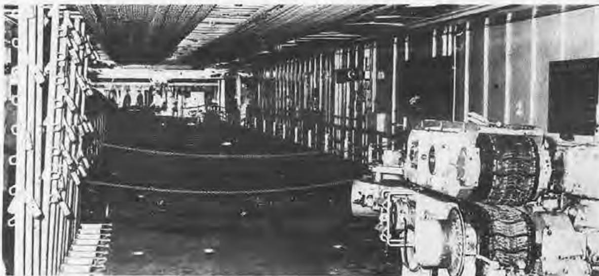
Above is a look at the main deck where cable is pulled from the storage tanks by specially designed linear cable engine at right. A pair of tractor-like treads grips the cable, moving it swiftly and evenly despite the varying depths at which the cable is being laid.
