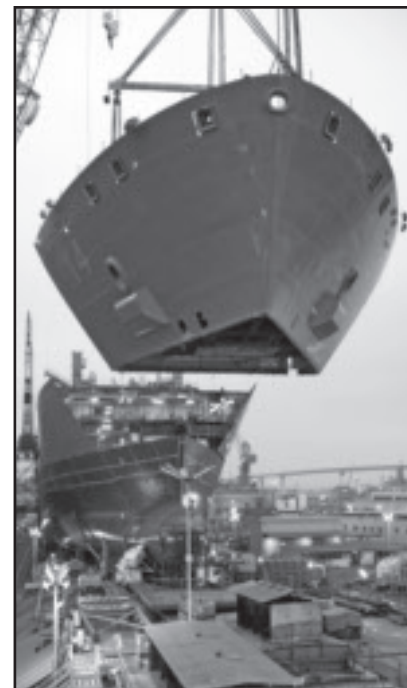
The 500-ton bow section of the USNS Cesar Chavez is hoisted in late October 2011. (Photo courtesy NASSCO)
