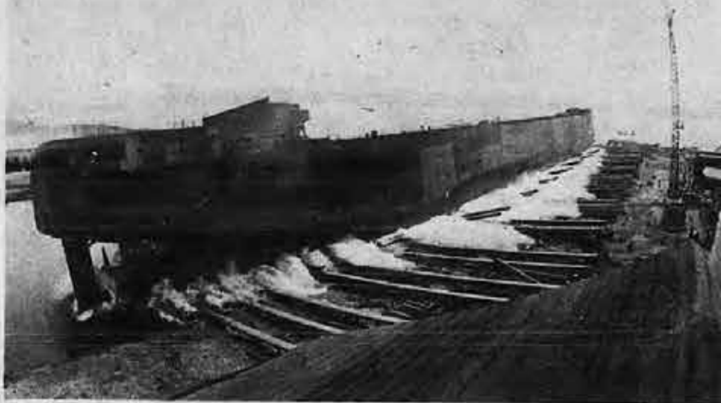
M/V Sam Laud is side launched in Sturgeon Bay, Wisc.
