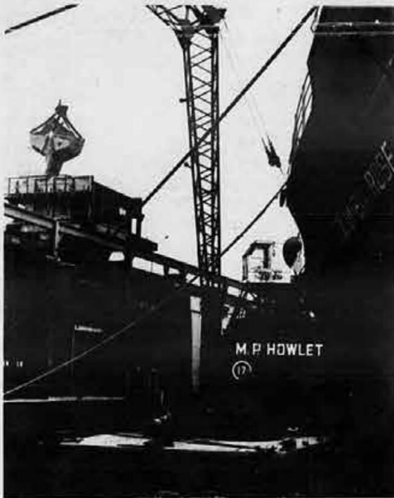
Bulk raw sugar is transferred from the hold of the *Columbia Rose* to a silo by a heavy-duty crane at the Richards Street dock in Brooklyn.
