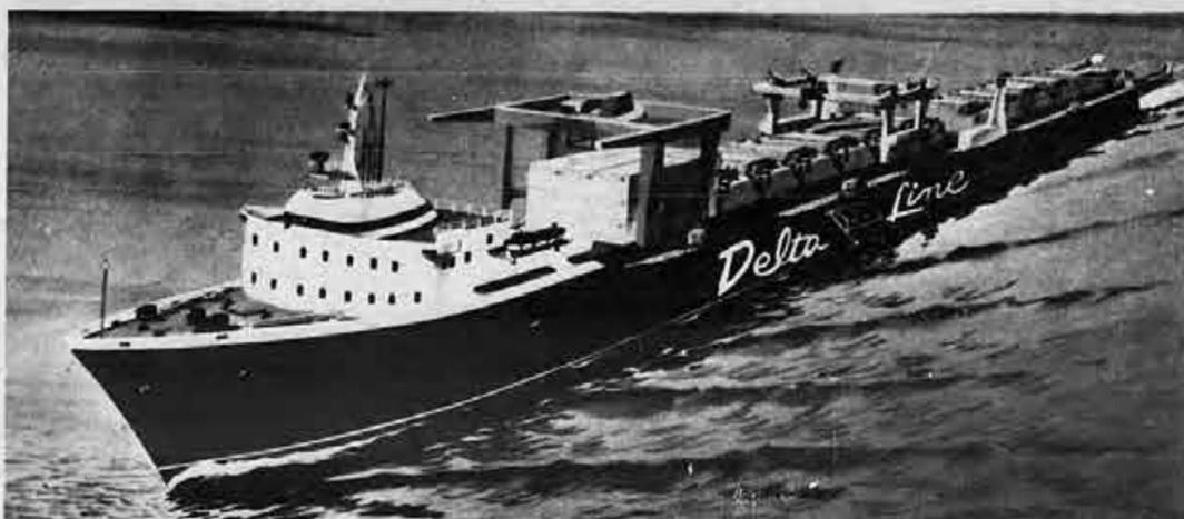
Delta Steamship Lines, Inc., has announced its intention to construct from one to six of these new LASH/Container cargo vessels which will be manned by SIU members. Each ship would be 772 feet long and would haul 64 barges or 1,500 containers—or a combination of both.
