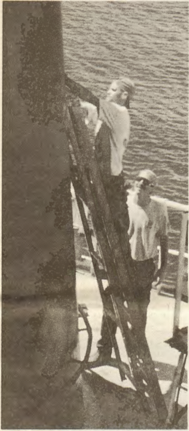
Shortly after signing aboard the Perseverance , ABs Justin Savage (on ladder) and Mark DePalma prepare to paint the stack while the vessel is docked in Yauco, Puerto Rico.
