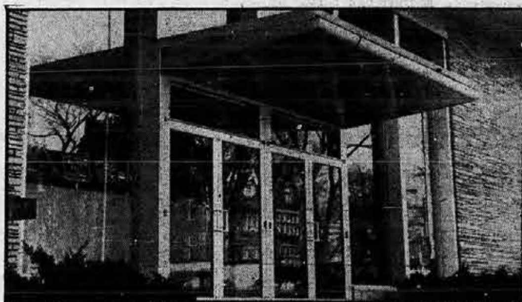
Done in modernistic style, UAW headquarters houses union administrative offices and more than two dozen divisions dealing with various functions, including education and community services.
