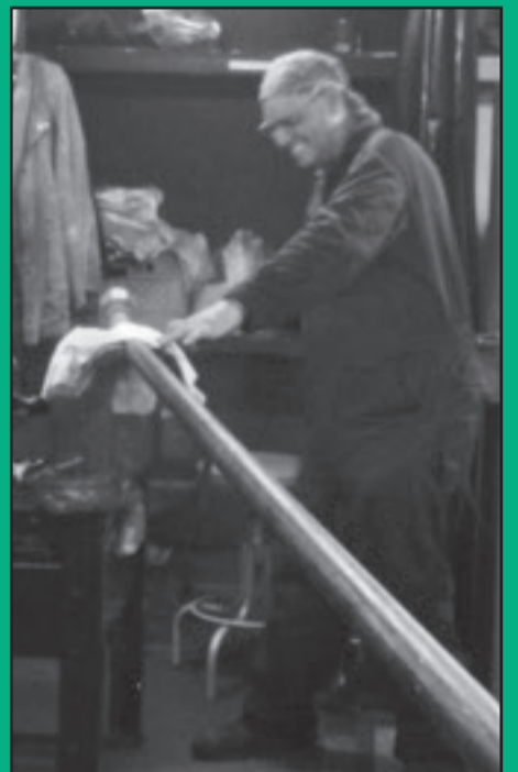
QMED George Rose paints drain pipes after welding.
