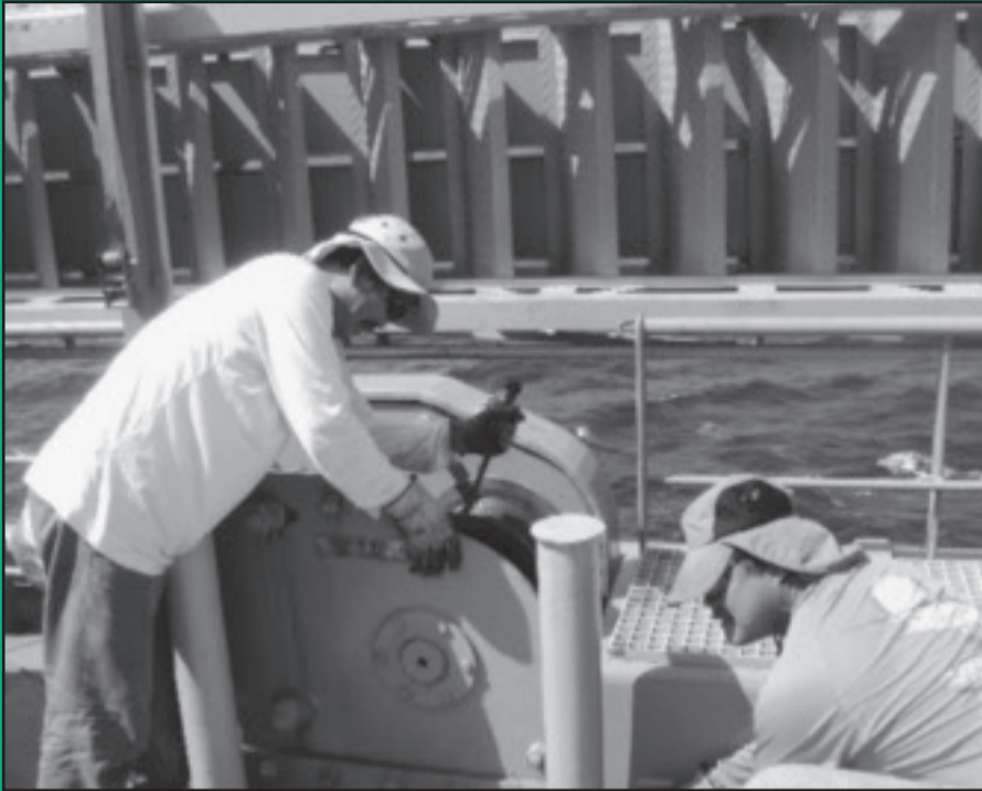
AB Xerxes Cunanan (left) and AB Randell Paredes work on cables.
