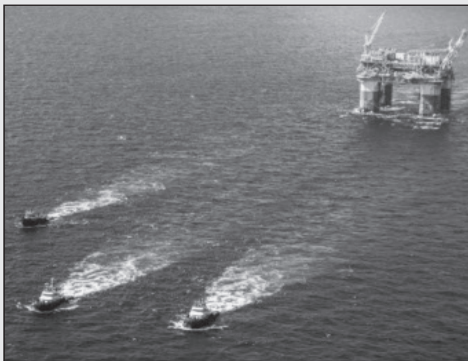
SIU-crewed tugs tow the equipment to its final location.
