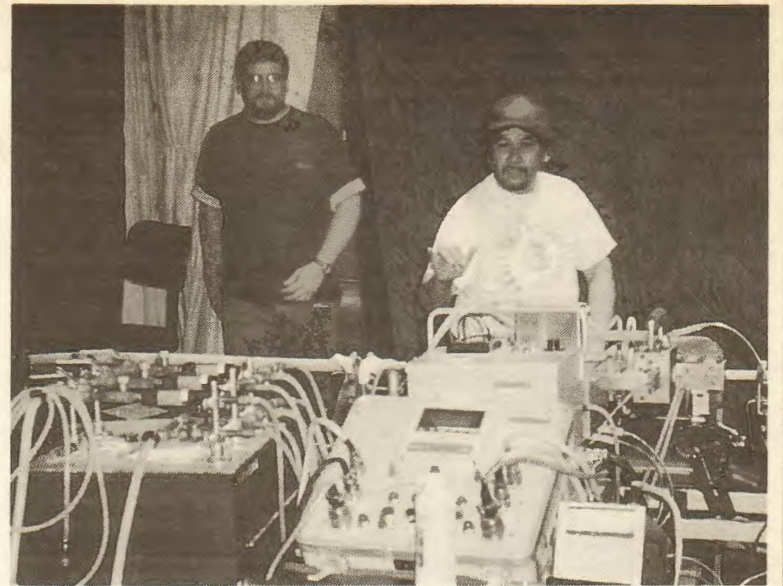
East meets West: The cables from Japan and the United States are spliced together. Joining the hair-thin fibers aboard the cable ship are a transmission technician (left) and Splicer/Joiner August G. Awong.
