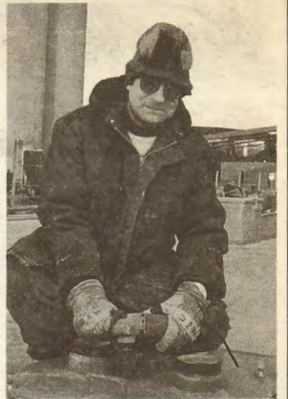
AB Michael Cushman cleans the inspection plates on the deck of the Medusa Challenger during winter layup.
