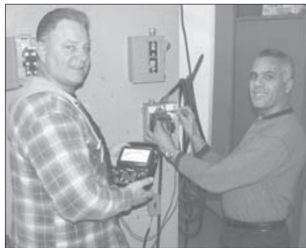
Norman Dauphin (left) and Hugo Infante perform a motor controller voltage check.
