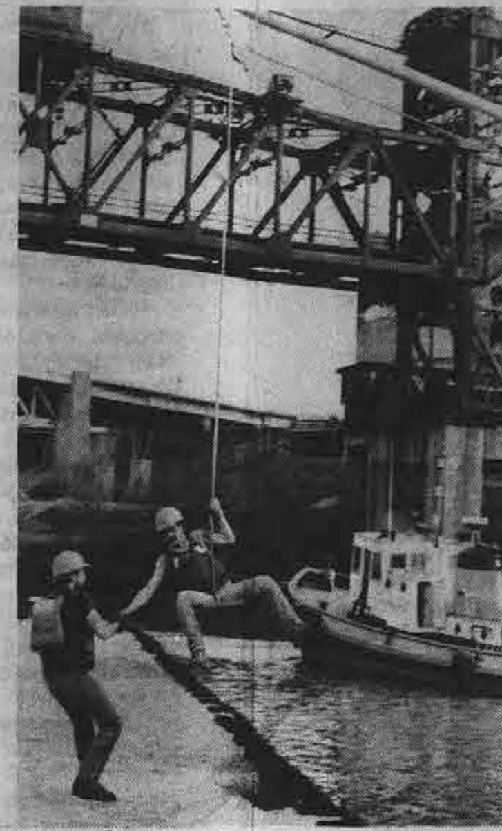
The fit-out on the Great Lakes is under way as deckhands Steve Halvaks (left) and Jeff Lalonde help tie up the Paul Thayer .
