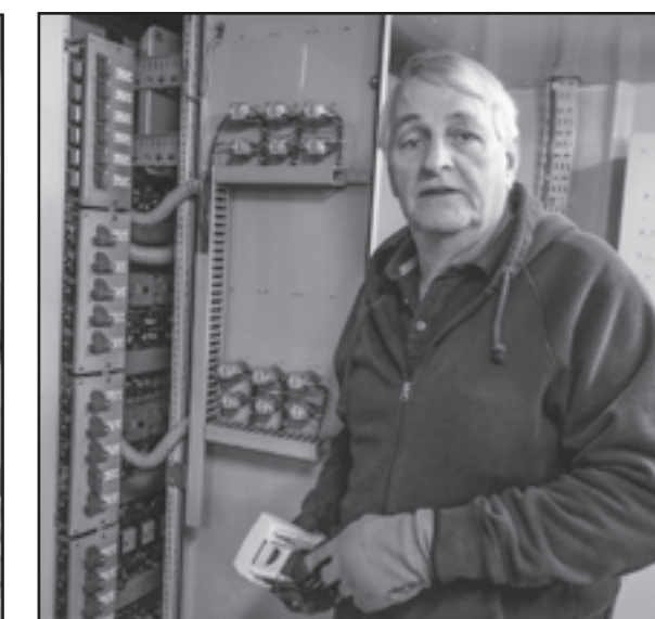
Electrician Dave Sexton Cape Washington
