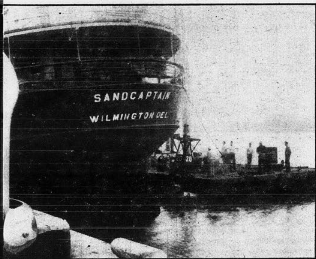
Front view of dredge was taken as a repair gang was working on pipeline which carries dredged materials into the watertight hoppers in ship's holds. Sandcaptain and two sister vessels, the Sandchief and Sandmate, last worked on land-fill job in Newark Bay during construction of famed New Jersey Turnpike. Venezuelan assignment is just the reverse of that job.
