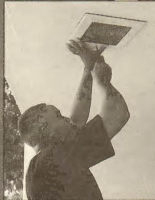
AB Ronald Webb installs light fixture in the new office.
