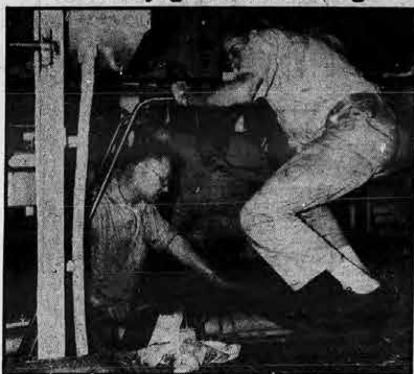
Candid shot catches a trio of licensed engineers working on a steam line below the operating platform on the Steel Voyager. Pictured (l to r) are engineers L. Symons, R. Maus and C. Reinhardt. SIU oiler A. Stakopoulos is partially hidden by Reinhardt. Engineers are members of the SIU-affiliated Brotherhood of Marine Engineers. The ship was in New York at the time.
