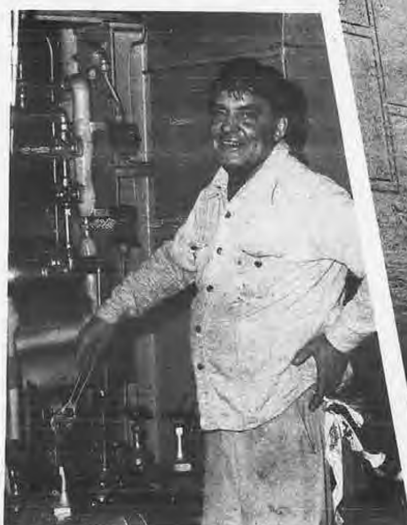
Oiler Edward Kwiatkowski has been shipping out for 35 years. Here he's checking out the evaporator which distills water for the boiler in the Cornelius ' engine room.
