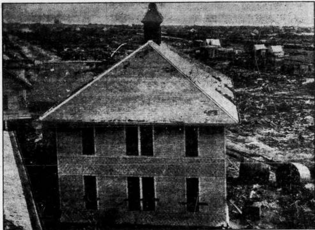
Hurricane winds carried this schoolhouse 600 feet from its foundations. To the rear are endless blocks that were swept completely clear of all homes. Destruction extended, Hiroshima-like, all the way to the horizon.
