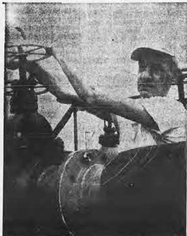
Tom Lowe lends assist on pumping job, opens valve so shore line can take cargo ashore.
