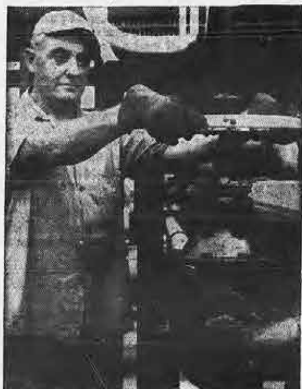
With lines connected up, Seafarer George McCurley gives valve a turn to start pumping.
