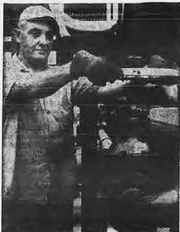
With lines connected up, Seafarer George McCurley gives valve a turn to start pumping.
