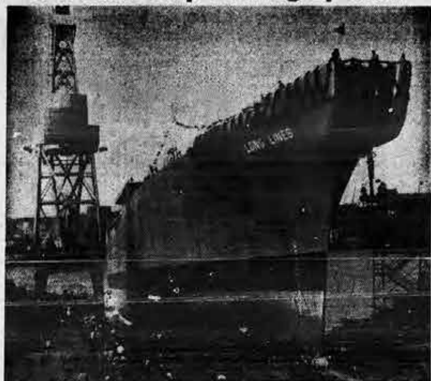
World's largest cable ship, shown at launching in Hamburg, is aptly named the Long Lines and will be operated by Isthmian with an SIU crew. Once the vessel is manned, crew will take part in shakedown training before heading out on first cable-laying voyage in the Caribbean. The odd-looking bow houses a reversible propeller which gives the vessel extra maneuverability.
