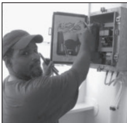
Electrician Christopher Eason
