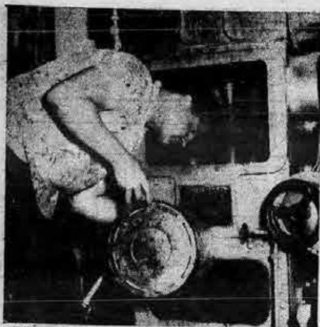
Oiler Al Saunders does a little oiling, namely, filling sump on manifold pump with lubricating oil.
