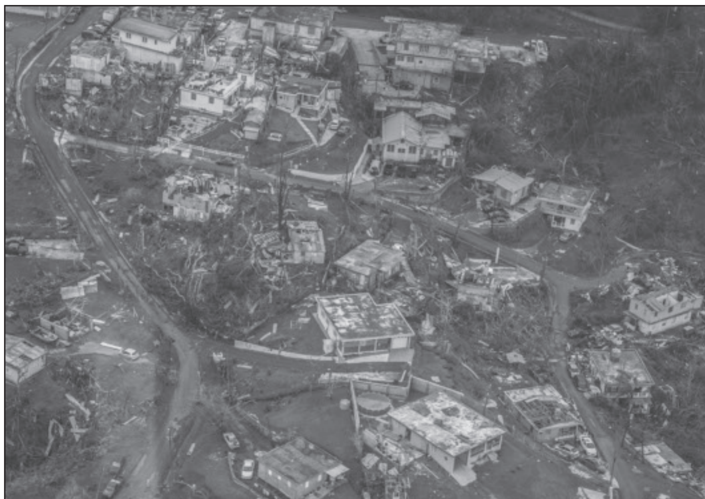
Some of Maria's destruction is seen in Aguadialla, Puerto Rico, on Sept. 24. (Photo by Kris Grogan, U.S. Customs and Border Protection)
