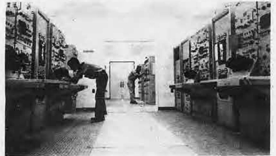
These two rooms of electronic equipment, valued at more than $430,000, are part of the Coast Guard LORAN transmitting station facilities at Grand Isle, La. This installation, and two similar ones at the cities of Galveston and Port Isabel, Texas, went on the air November 1 to bring all-weather, precision navigation to the entire Gulf of Mexico.
