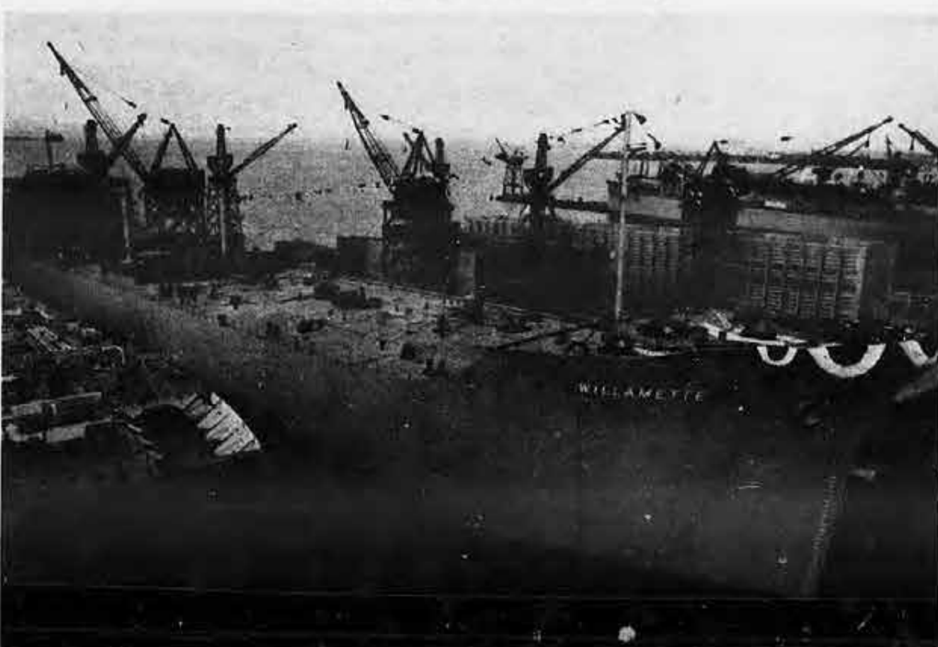
Latest addition to fleet of SIU-contracted Bulk Transport, was 37,250-ton tanker S. T. Willamette, recently launched at Bethlehem Steel's Sparrows Point shipyards. Named for Oregon's Willamette River, vessel is first of two of this class constructed for Bulk Transport. The vessel has a cruising range of 12,000 miles.
