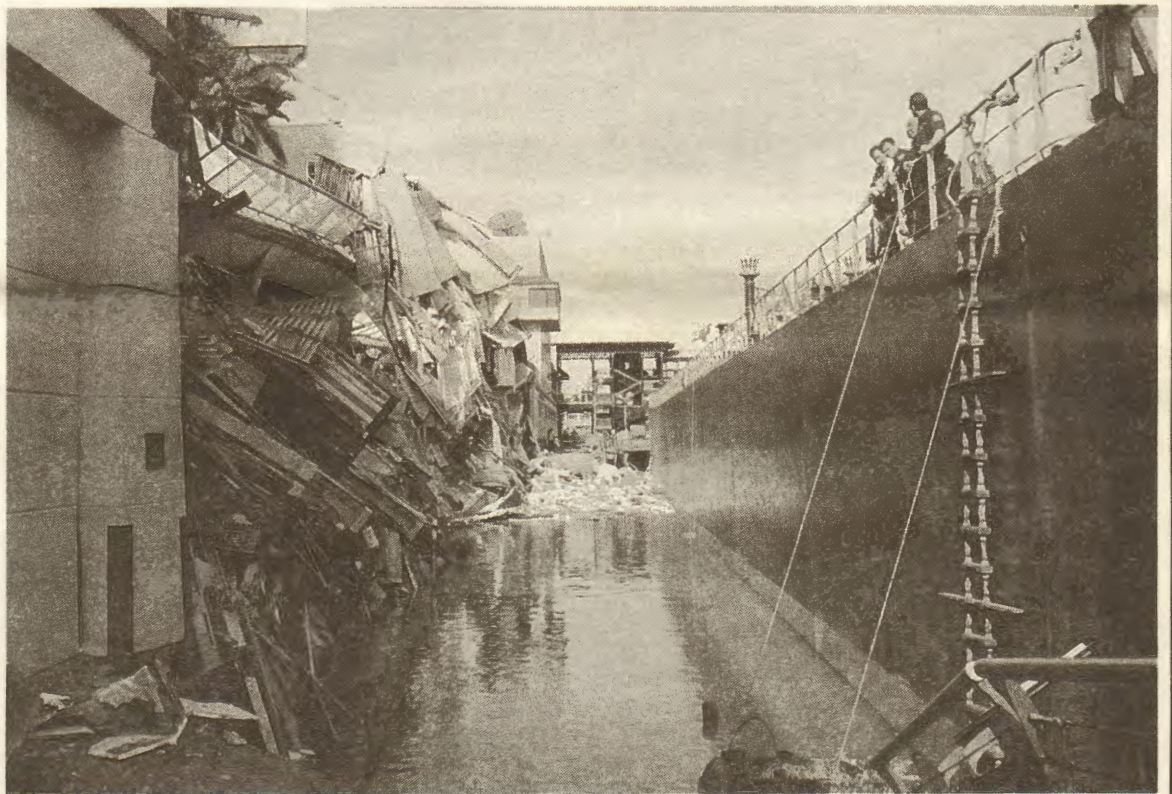
The runaway-flag Bright Field , owned by Cosco Shipping of Hong Kong, crashed into the Riverwalk Marketplace pier in December 1996 after losing engine power. Investigations into the accident—which resulted in more than $20 million in shore-side damage and injured approximately 100 people—concluded that Cosco is primarily to blame.
