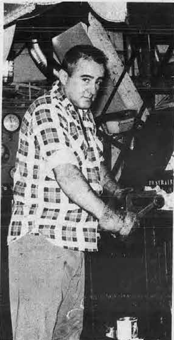
Fireman-watertender John Petino changes tip of burner in the engine room.
