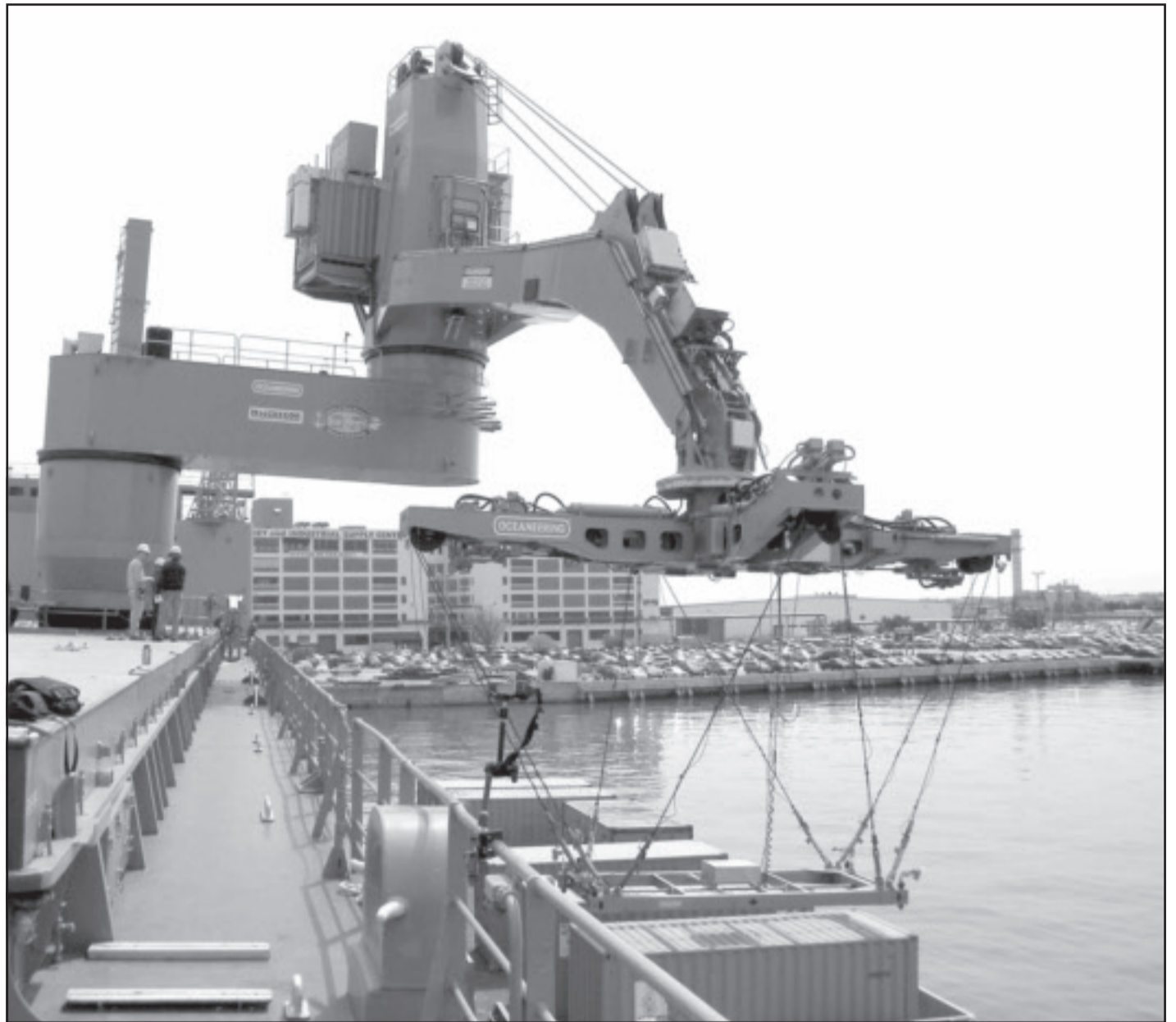
Office of Naval Research personnel test their Large Vessel Interface Lift-on/Lift-off (LVI Lo/Lo) crane at the U.S. Naval Station in Norfolk, Va. The demonstrator crane, which has been temporarily installed on the USNS Flickertail State uses motion-sensing technology to control standard 20-foot containers in all six degrees of freedom. (U.S. Navy photo)
