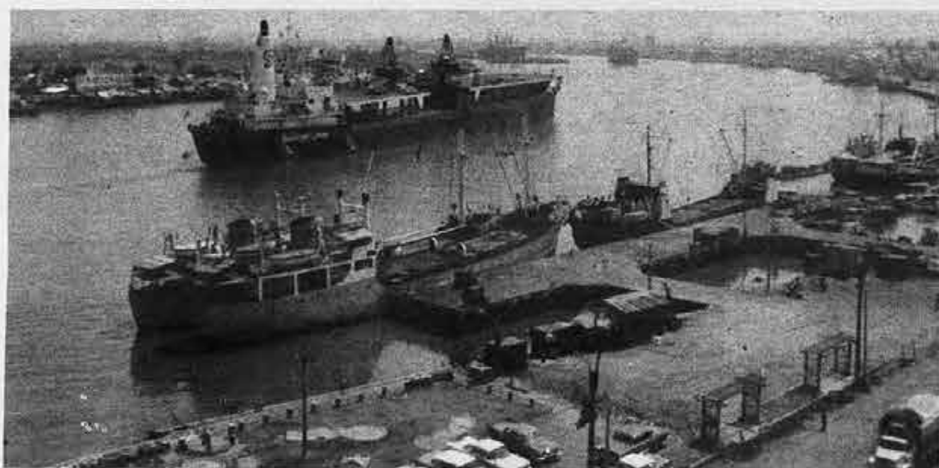
Seatrain Puerto Rico heads down the twisting Saigon River to sea. There are many sharp zig-zags and "sticky" bends to be negotiated when "running" the river. The swift current is also a test of a pilot's nerves.
