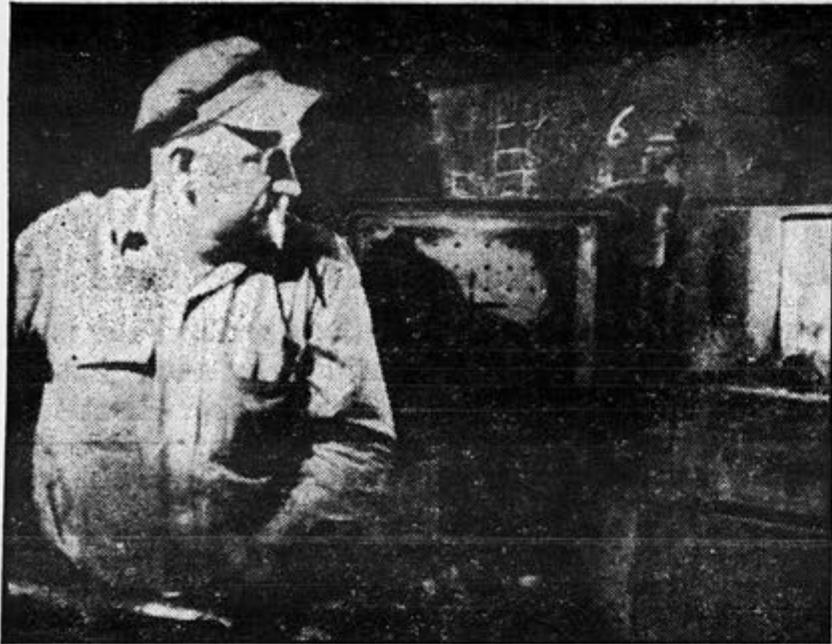
Fireman Bishop Creech of the SIU Great Lakes District throws bucketful of coal on fire of the Huron, a bulk carrier. Huron was slated for conversion to oil, but rising price of fuel has kept her on a coal diet.
