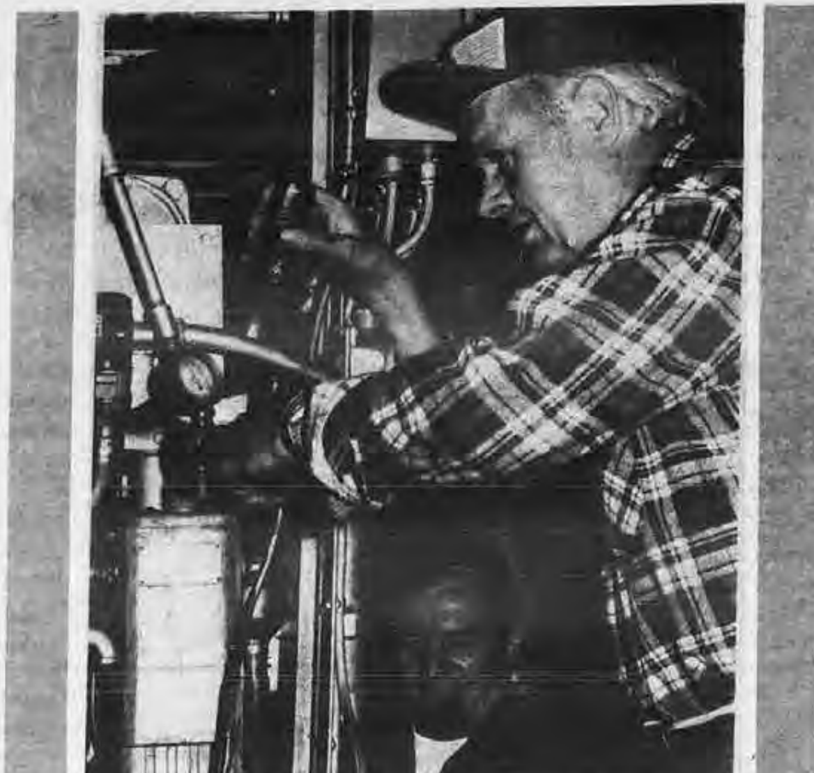
On the Great Lakes Towing tug Arizona , SIU Boatmen Rudy Jadrich and William Blanchard make some routine engine repairs.
