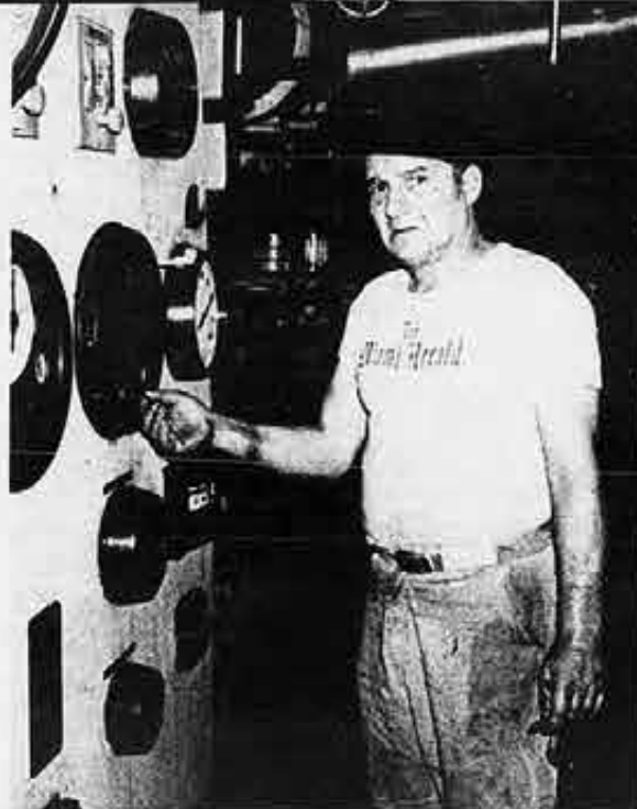
Fireman Ignatius Salerno checks panel board in the engine room aboard the Tampa . Brother Salerno joined the SIU in the Port of New York in 1961.
