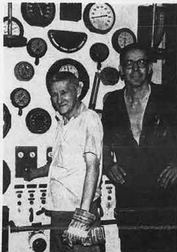
Fireman C. White and Oiler R. Vance in the engine room of the DeSoto while in the port of New Orleans.
