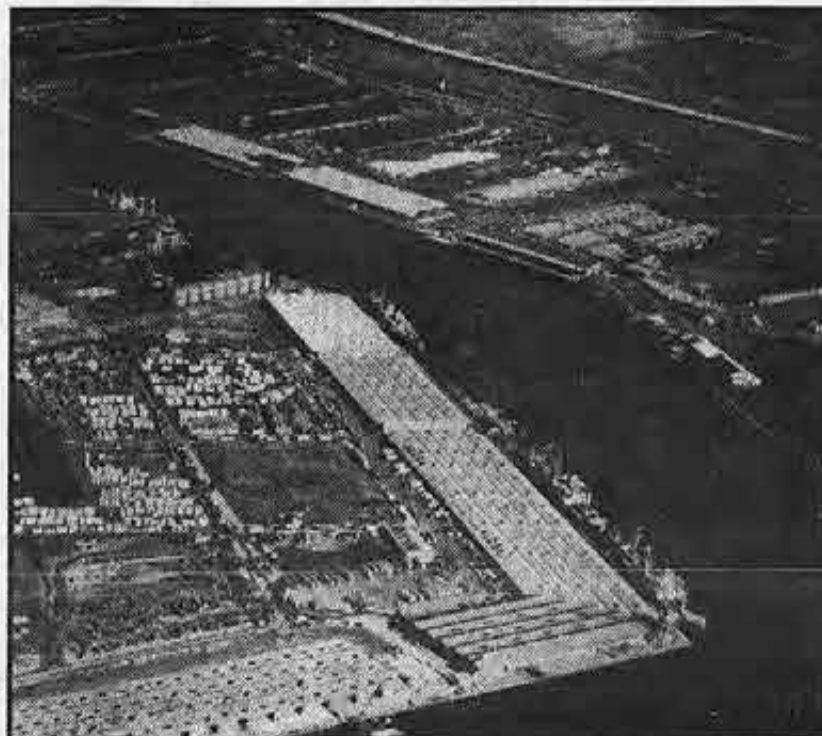
Aerial view of new Alcoa Steamship terminal at Port Newark, NJ, following shift from Brooklyn piers the company formerly occupied. Both Alcoa and Waterman-Pan-Atlantic, located nearby, now have all terminal operations in New York area concentrated at Port Newark.
