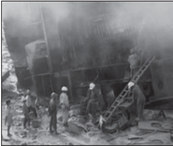
An explosion and fire occurred in the hull of a tanker, killing, burning and maiming numerous workers.
