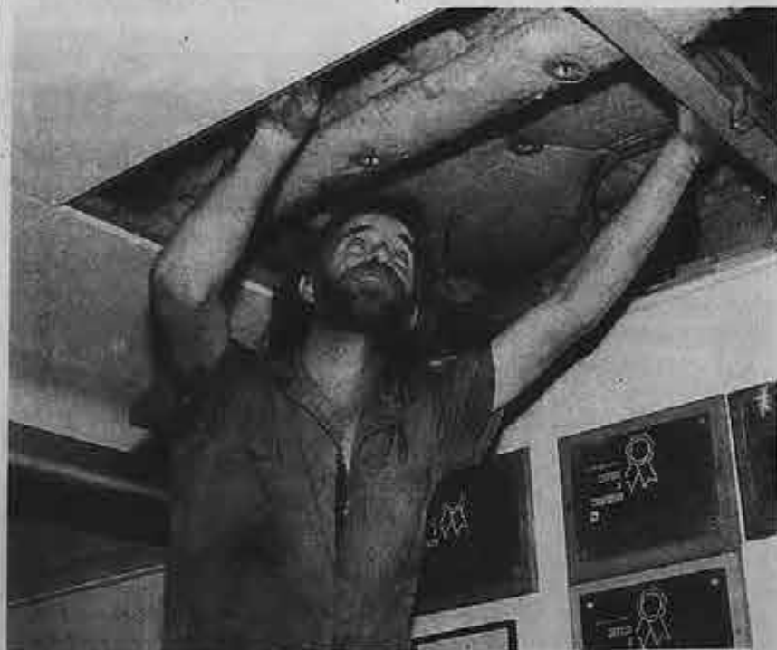
Electrician Robert Adams runs a cable through the overhead.
