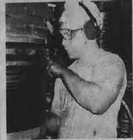
Cleaning a piston in the engine room is DEU Mike Morgan.
