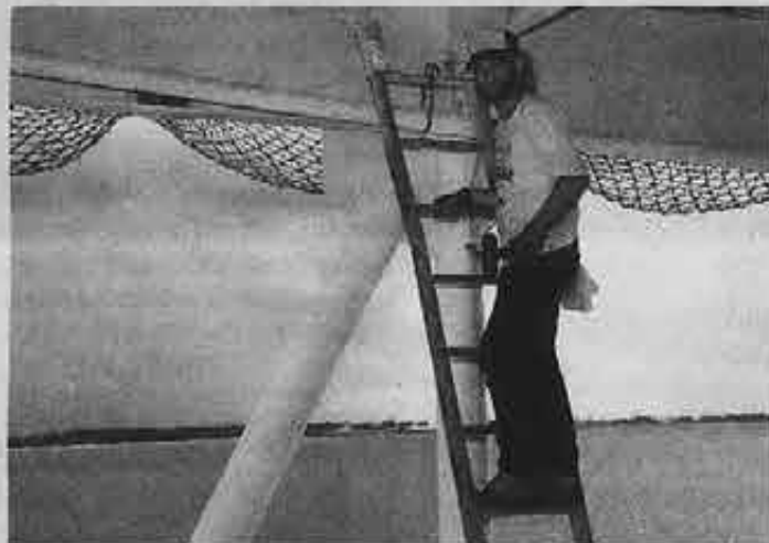
To unclog the drain pipes under the helicopter landing pad, AB Norman Tourtellot has to bang on them.
