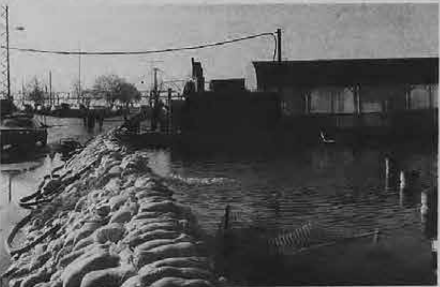
Sandbags try to keep the Mississippi River from flowing into the parking lot of the Alton Belle Riverboat Casino. The pilings nearly underwater on the right are the normal banks for the river.
