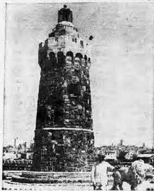
The traditional lighthouse, like this one in San Francisco, is constructed of stone in a cone shape. However, modern construction techniques and sophisticated instrumentation have changed lighthouse design drastically—shown at left below.
