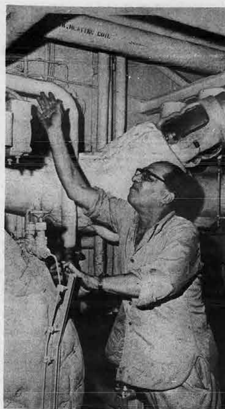
Seafarer Henry Delprado, who sails as QMED, tends to routine duties in the ship's automated engine room.
