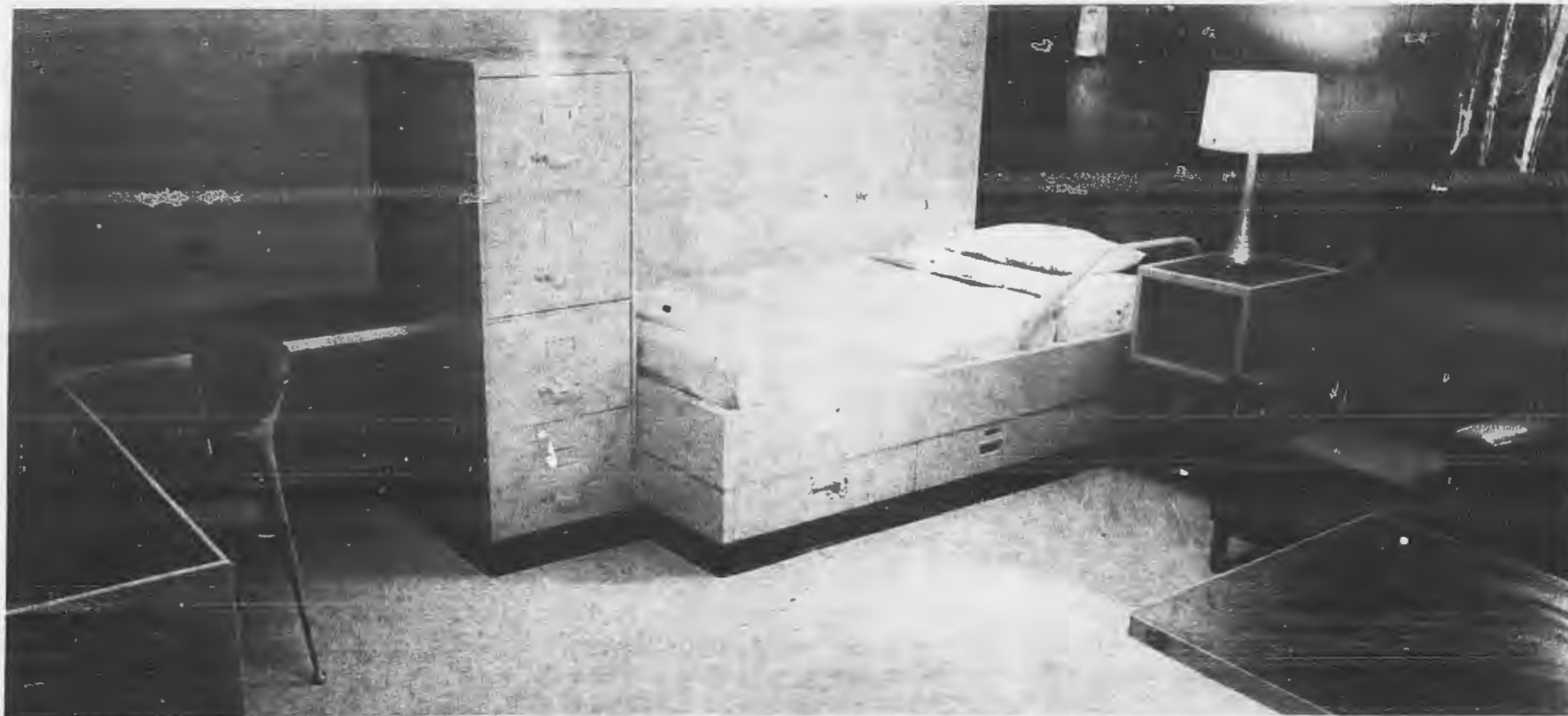
The Bosun's quarters on the ULCC.
