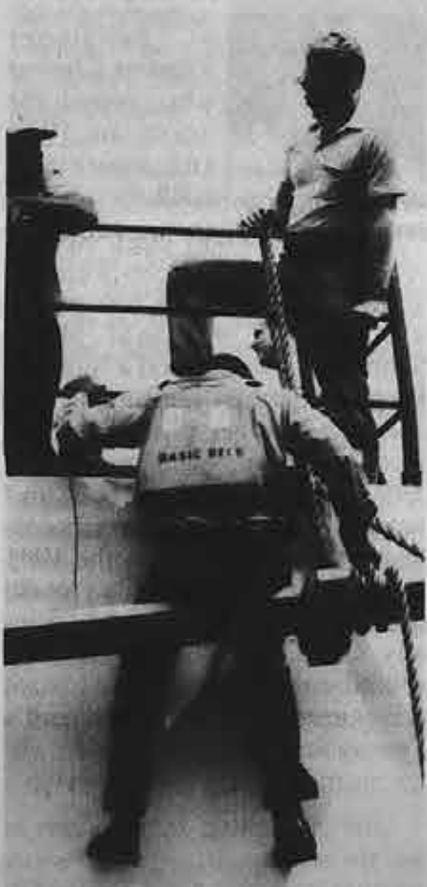
Recertified Bosun Jeremiah Harrington (standing right) instructs trainees at the Lundeberg School how to use a stage for painting and chipping.
