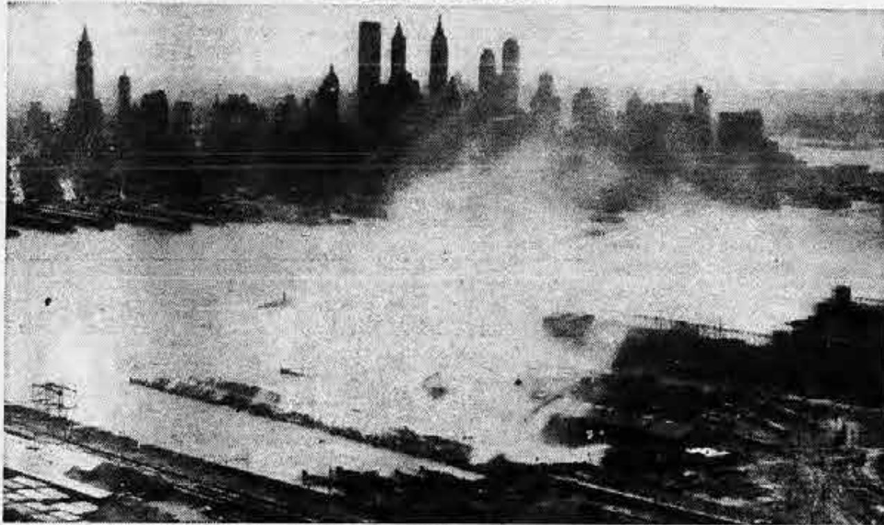
Pier Fire. Aerial photo shows smoke still pouring from piers of the SIU-contracted Pennsylvania RR in Jersey City. SIU Railway Marine Region members gained praise for heroic action during the blaze which gutted piers and equipment. (See Page 2.)
