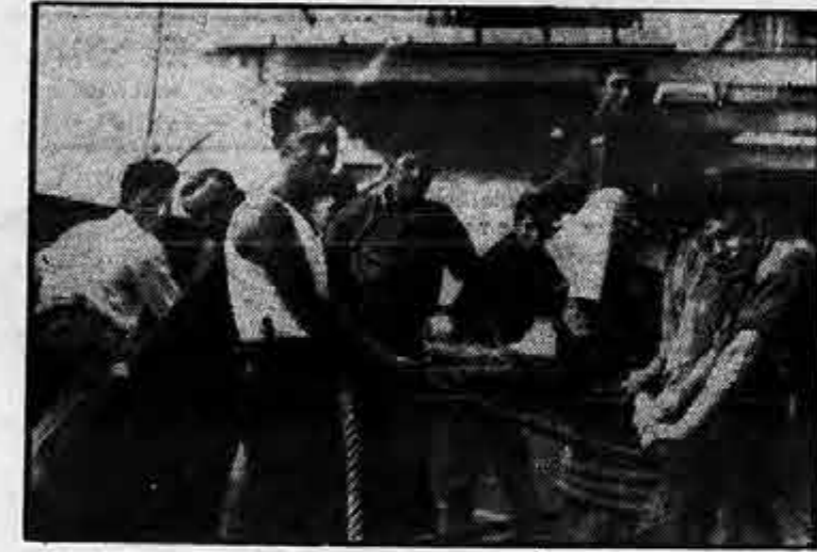
Crew works the capstan to the accordion's tune.
