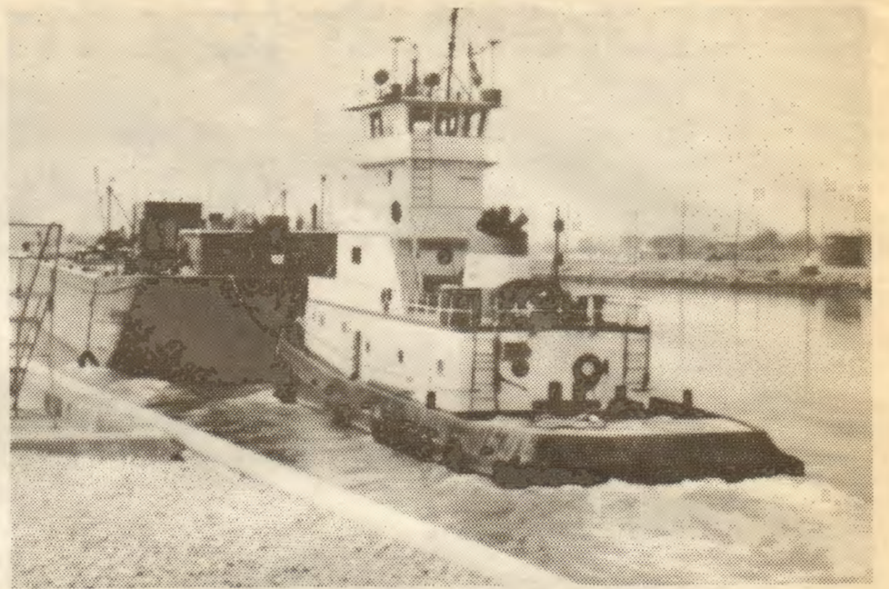
Boatmen aboard the Interstate Transport tug Schuykill head down river from the refinery.
