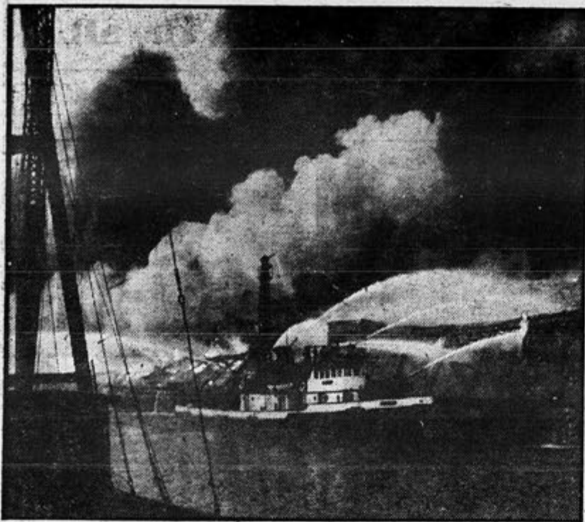
Dense smoke almost blots out scene as NYC fireboat pours water on flaming Luckenbach 35th Street pier. Blast rocked SIU headquarters and surrounding area.
