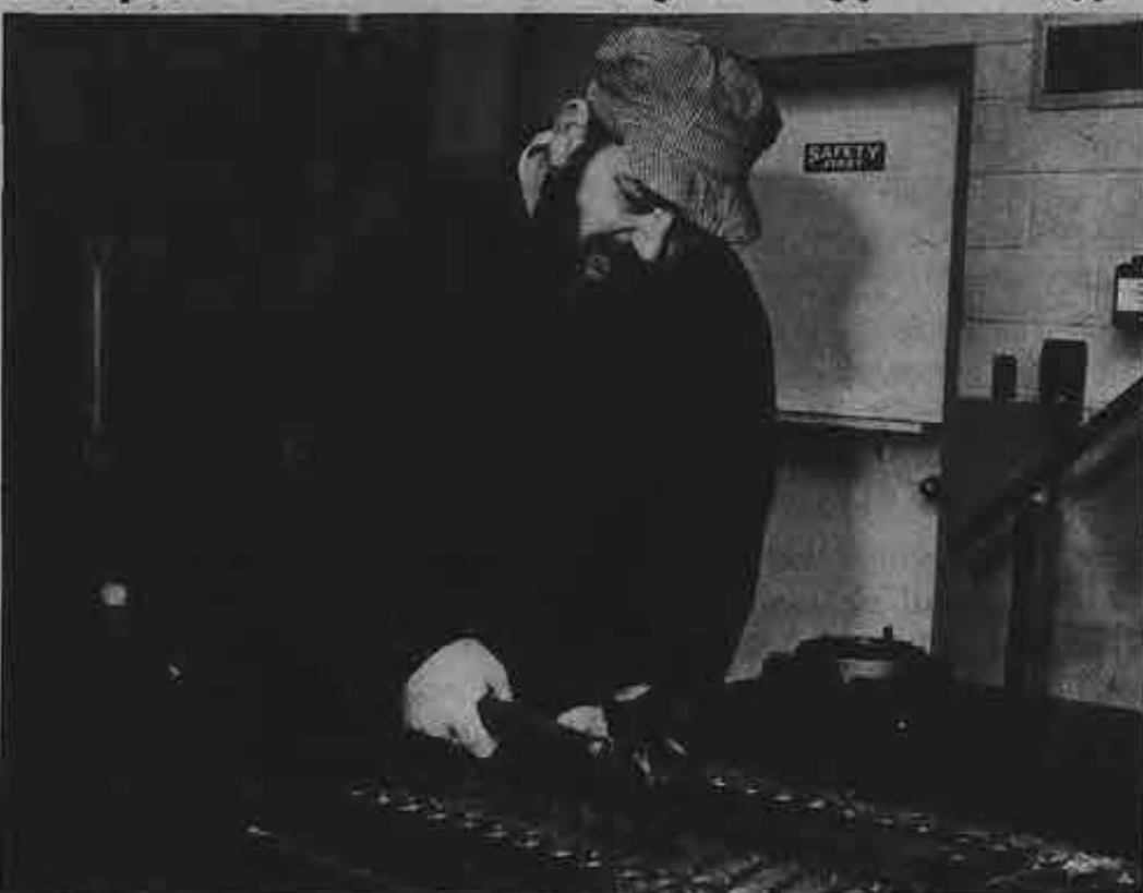
Seafarer Maynard Baker makes final adjustments on a repair job he was doing on a typical conveyor belt. Maintenance and repair of conveyor equipment aboard the big self-unloaders that ply the Great Lakes is an essential skill.
