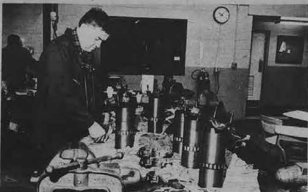
Hands-on training is an integral part of the upgrading programs at the Seafarers Harry Lundeberg School of Seamanship. Here, Seafarer Michael Burns checks connecting rod bearings as part of the Diesel Engine course.
