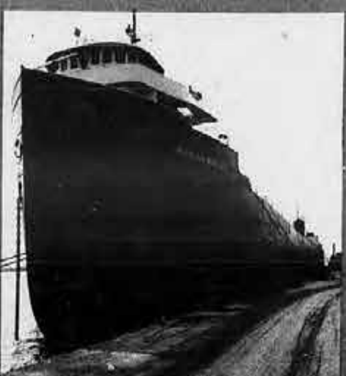
Buckeye Monitor's bow section towers high above dock at Detroit where the vessel was prepared for new season.
