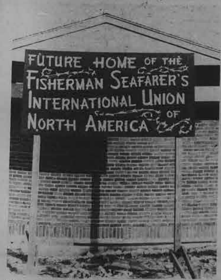
Next year's religious procession will pass right by the SIU's new Gloucester Hall, now under construction.
